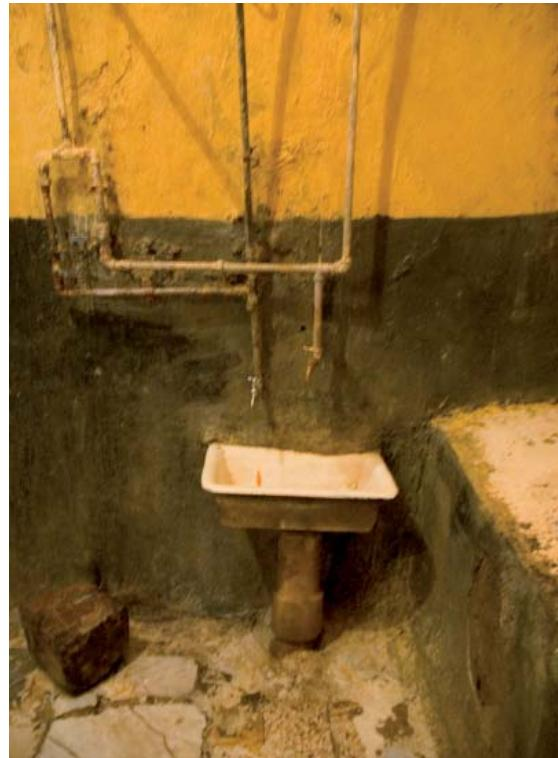
Figure 4 Poor Quality Water Pipes Insensitively Introduced in the Hammām. (Source: Sibley, M- AHRC funded project: Historic Hammāms of North Africa@June 2007).
